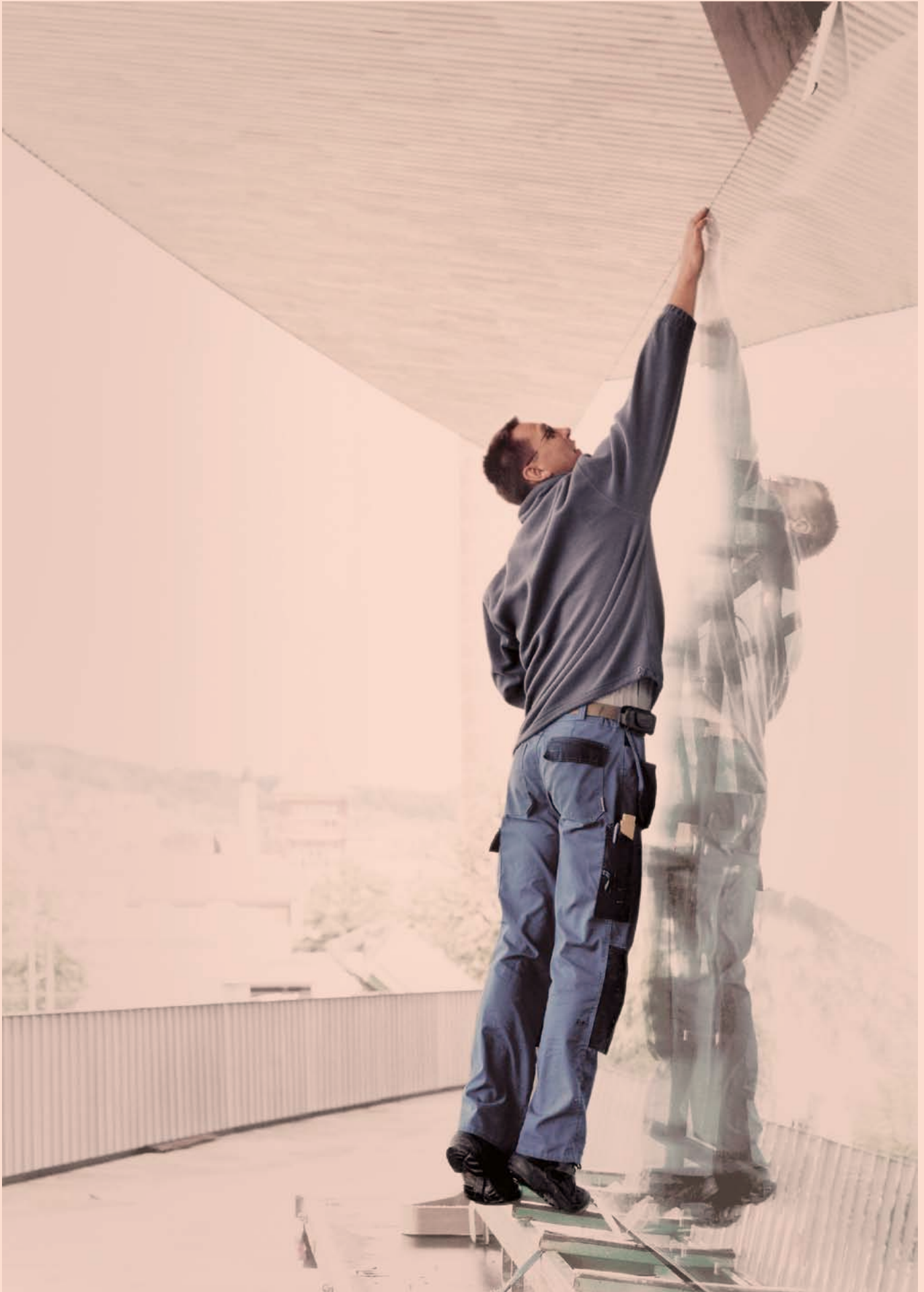
Installation by local partners.
