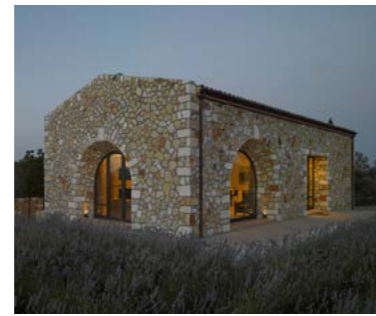
Project: GIESE Architect: Andrew Batey
