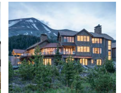
Project: LONE MOUNTAIN HIDEAWAY Architect: JLF Architects
